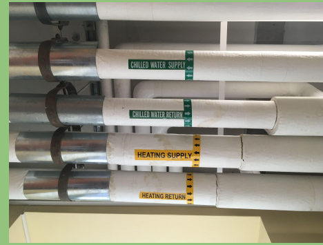
Insulated pipes
