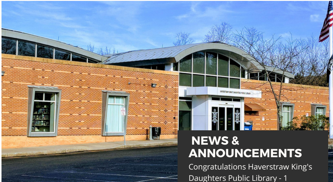
Exterior of Haverstraw King's Daughters Public Library Photo Credit: HKDPL Facebook page
