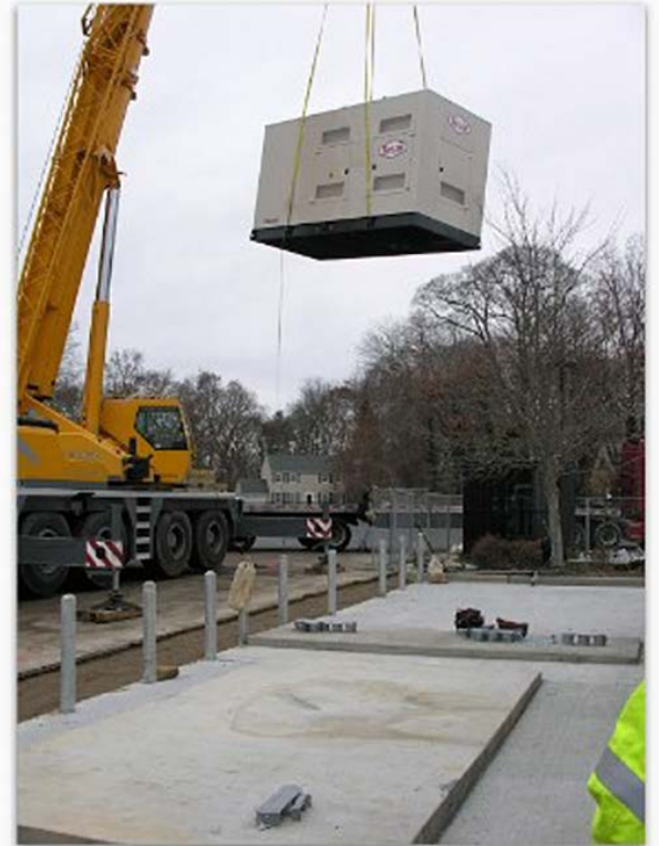
Pictured above: Installation of the library's backup generator
