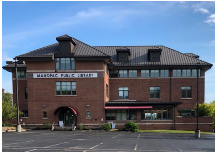
Mahopac Public Library considered a roof and ground-mounted solar installation
